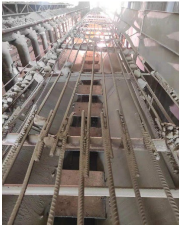
Technological transformation of belt conveyor hopper
