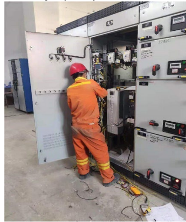
Installation of frequency conversion control
