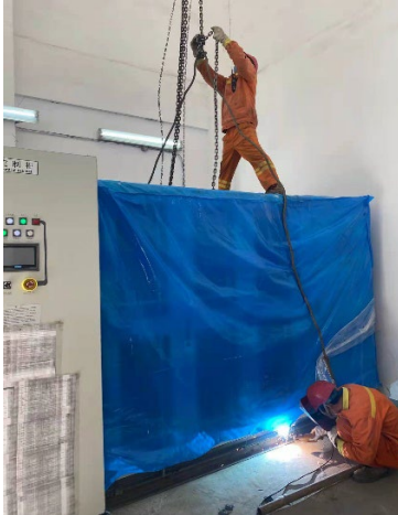
Replacement of kiln tail inverter
